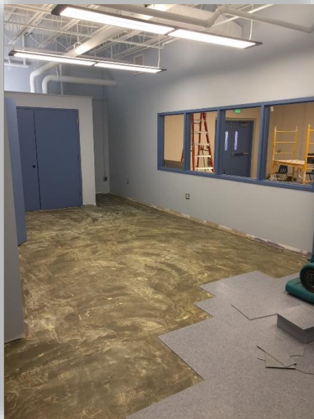
Installation of the floors in the STEM Center.
